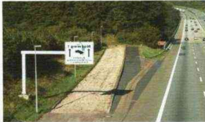
Gambar 73 Lajur Tambahan ( Service Road )
