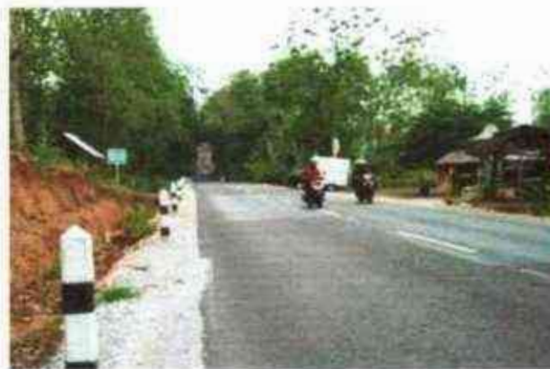
Gambar 48 Delineator Beton
